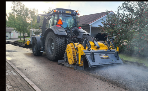
RC90 On-site asphalt recycling
