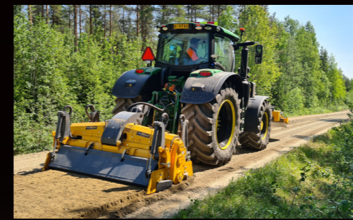
RC65 Gravel road maintenance
