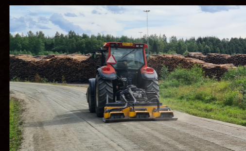
MPC-375 Gravel road maintenance
