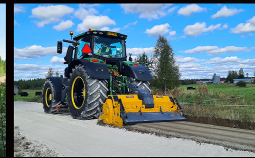
RC65 Stabilization and mixing of binders
