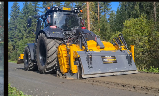
RC90 Gravel road maintenance
